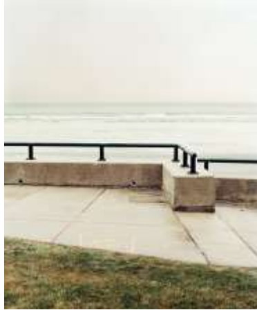
David Greer Hibernia Atlantic transoceanic cable landing, Lynn MA
