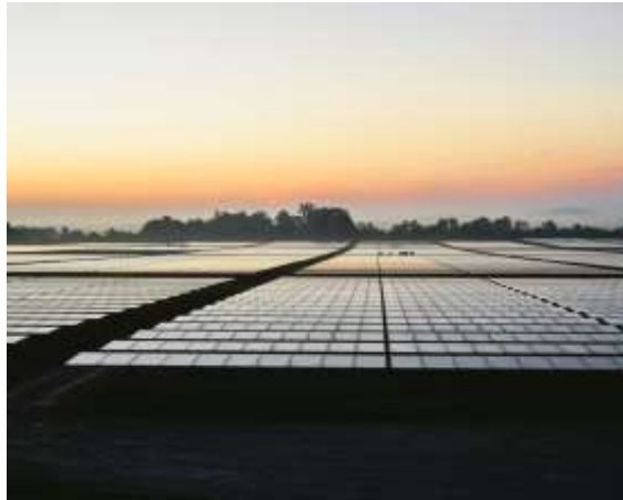
David Greer Apple's 14MW solar array, Maiden NC
