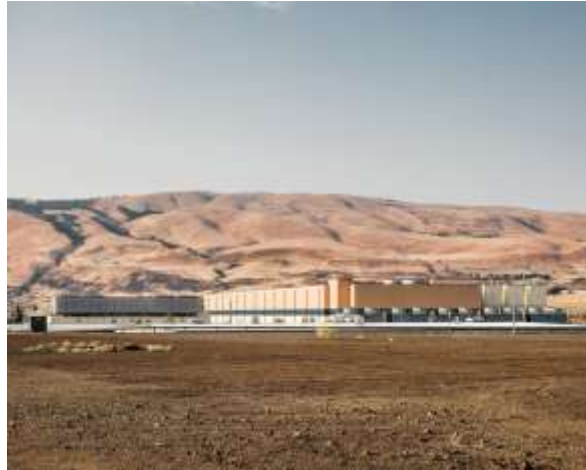
David GreerGoogle data center, The Dalles OR
